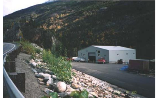
Figure 10: Skagway's material handling and recycling facility with their Thermal Oxidation System.
