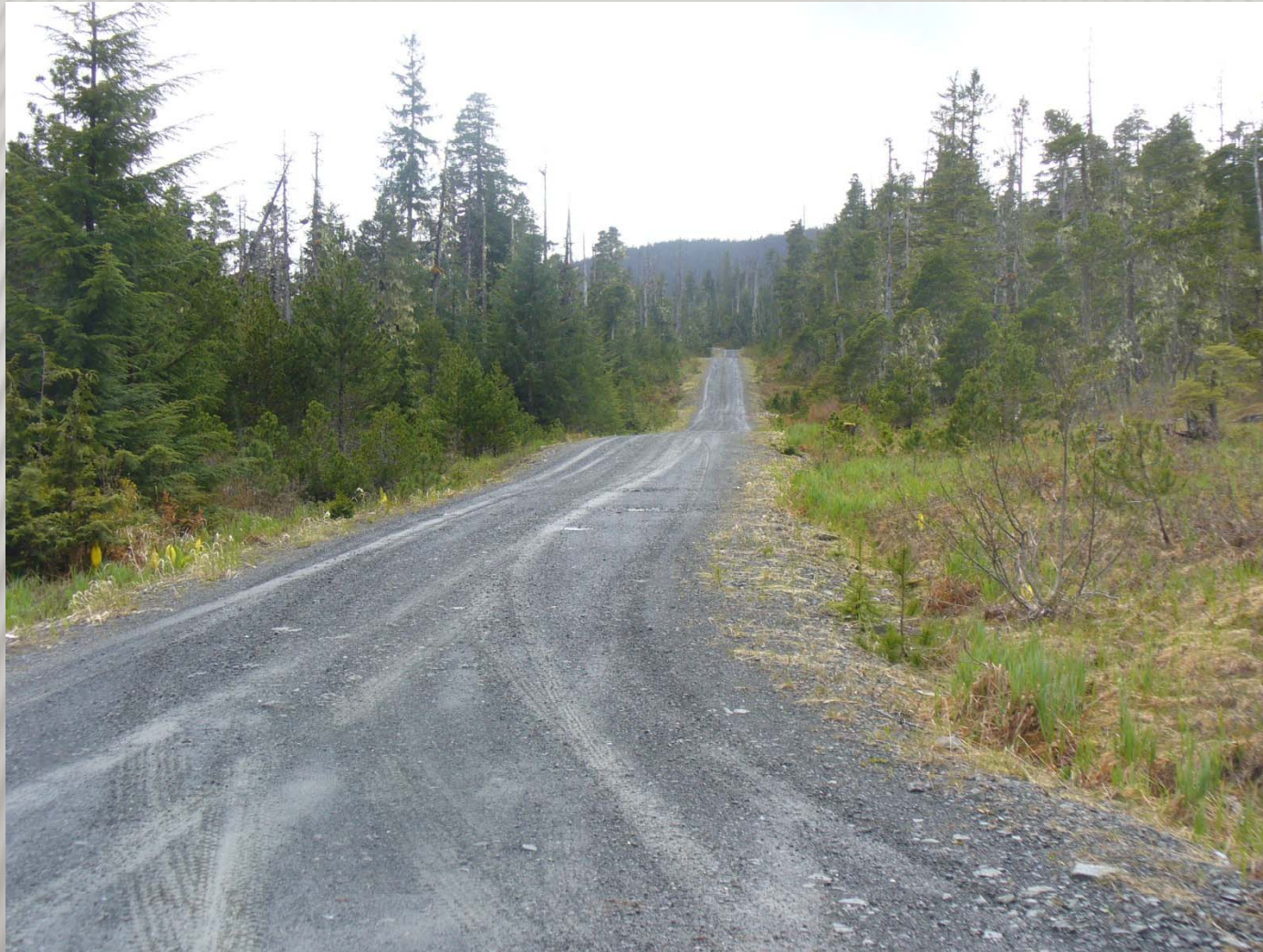
Typical USFS Road on Kupreanof Island
