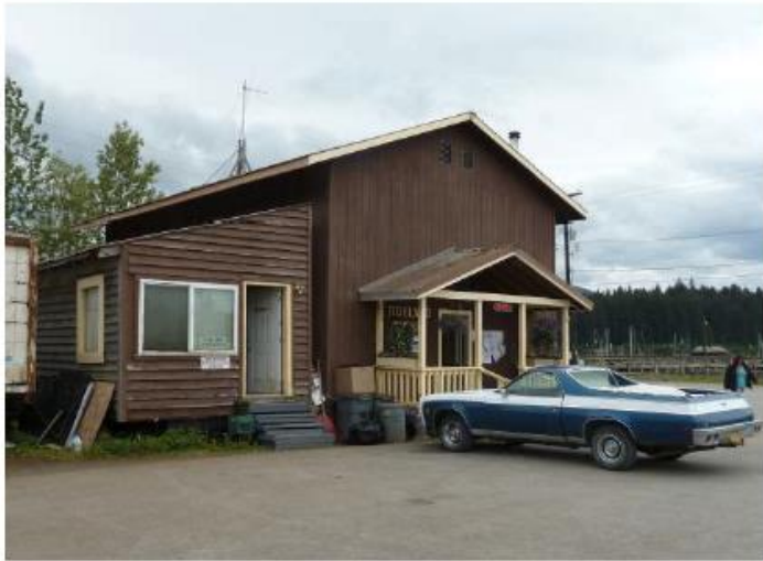
Level 1 Targeted Commercial Energy Audit Tideland Tackle Store
